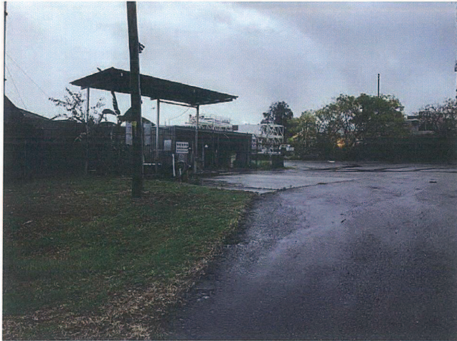
Photo 3 Sullage pumping station on the site
