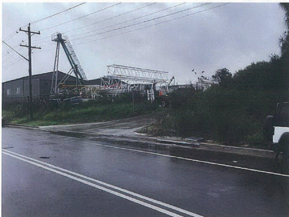
Photo 4: Sullage pumping station on the site
